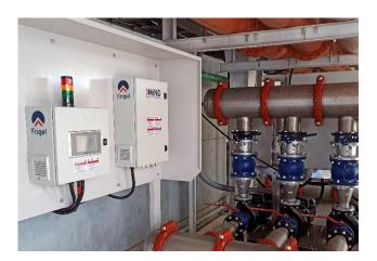
It allows to observe and manage the working parameters of the machines through a multifunctional user interface, both locally and remotely, with an easy-to-use web interface. **MiND** is able to provide customers with a perfect supervision and maintenance tool for all Frigel equipment.
